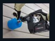
Siding panel drilling with core hole saw (ø160 x 16mm)
